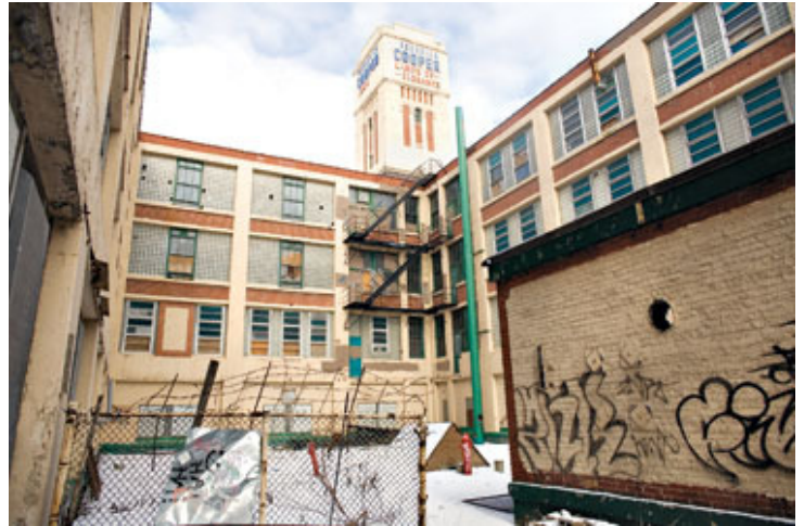
The shuttered Frederick Cooper Lamp Factory, 2500 block of W. Diversey, will be converted into a green business incubator in 2008, providing 300-400 jobs.
